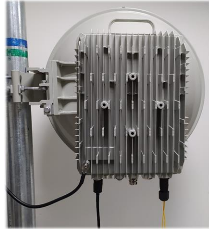
Dual-channels in each subband using dual polarization (XPIC) with OMT
